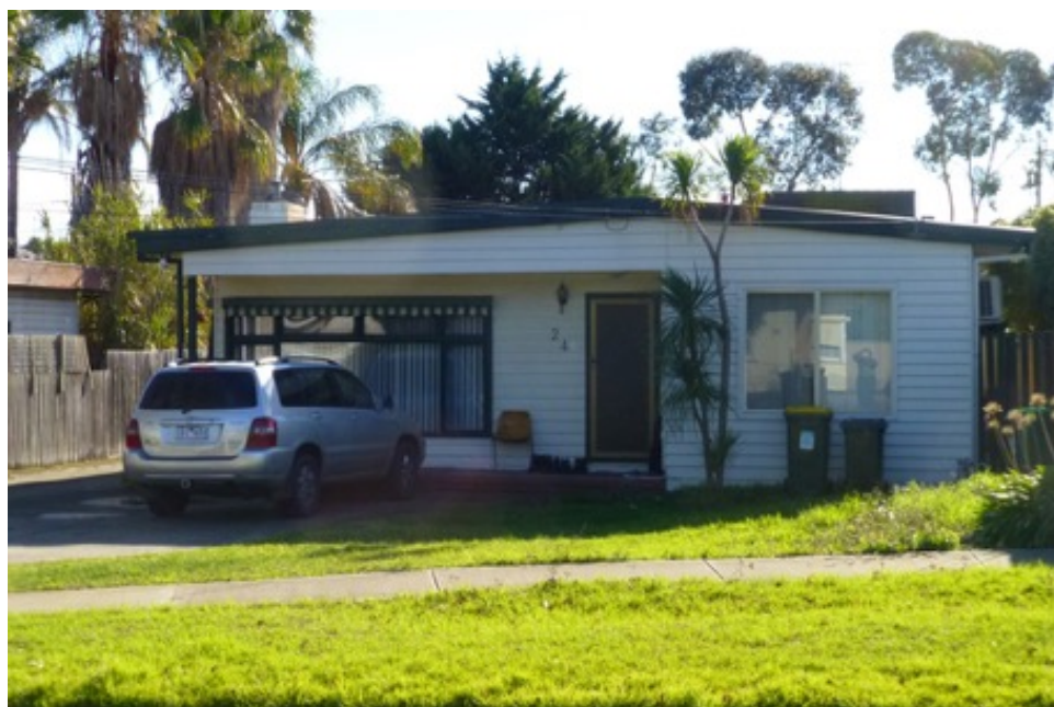
Figure 27 Group 3 half-house in Shirley Street. Source heritage Alliance 2019
