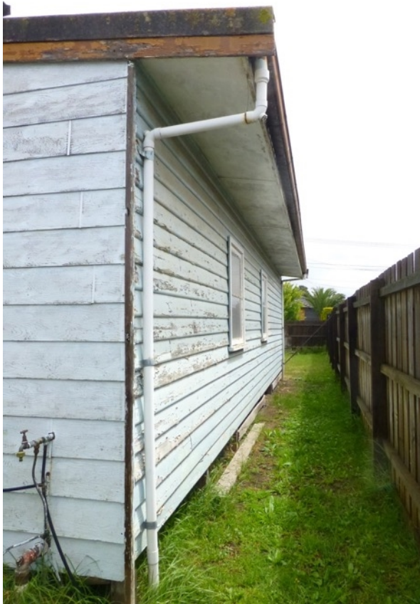
Figure 21 Eastern façade showing bull-nosed timber weather-boards. Source, heritage Alliance
