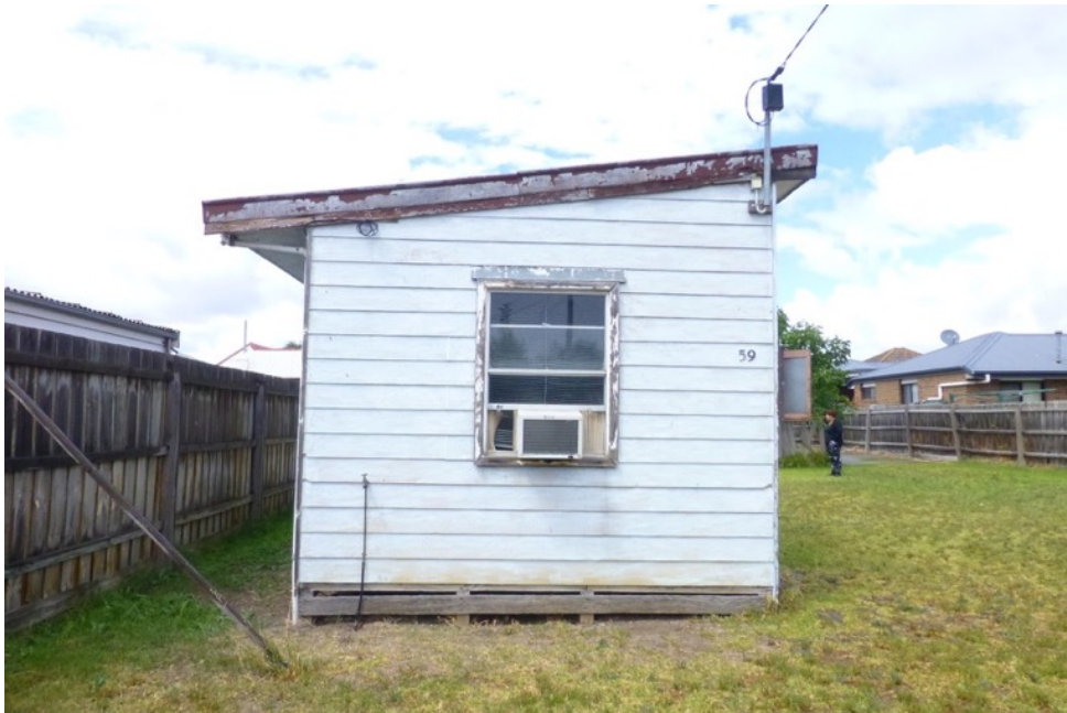
Figure 19 Northern façade facing George Street showing compressed fibre cement sheet boarding and metal sash window. Source, heritage Alliance
