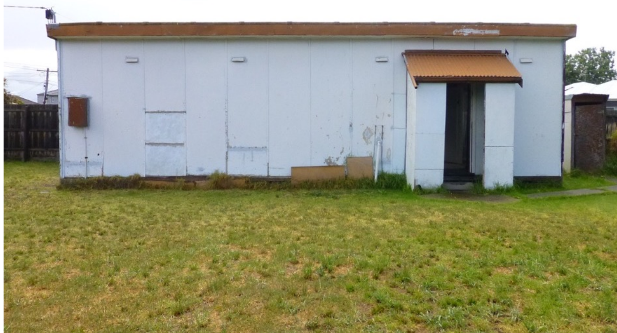
Figure 18 Western façade 59 George Street, St Albans. The principal façade is made of a series of asbestos cement sheets on a timber frame. To the right hand side is the only door to the house enclosed by an asbestos cement porch and metal roof. All photographs taken 26 November 2019. Source, heritage Alliance
