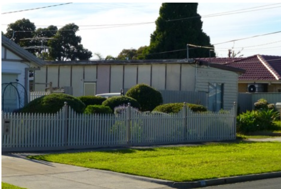
Figure 23 Group 1 half house in Shirley Street. Source, heritage Alliance 2019
