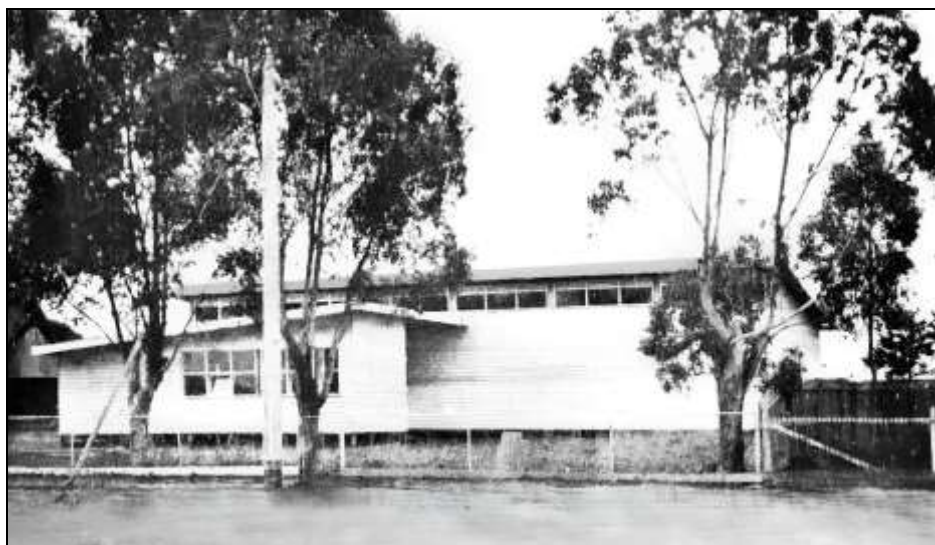
St Alban The Martyr Church Hall and Kindergarten 1960s
