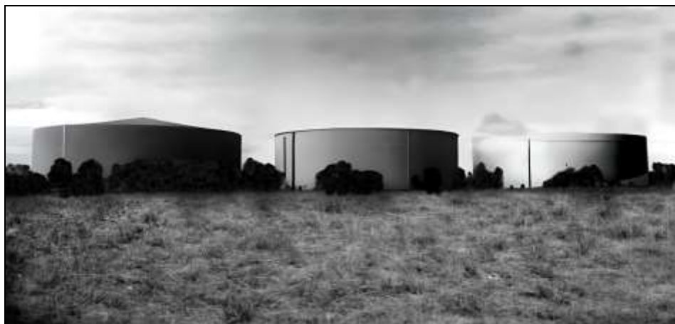
Water tanks in Taylors Road 1970s c/- St Albans First 100 Years
