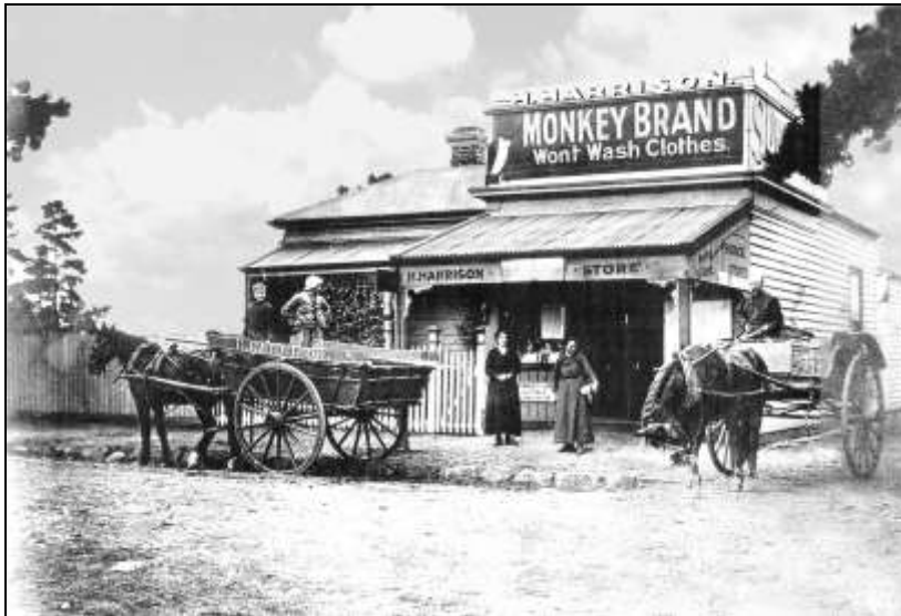
Weatherboard house & shop in Main Road West near Amy Street 1920s
