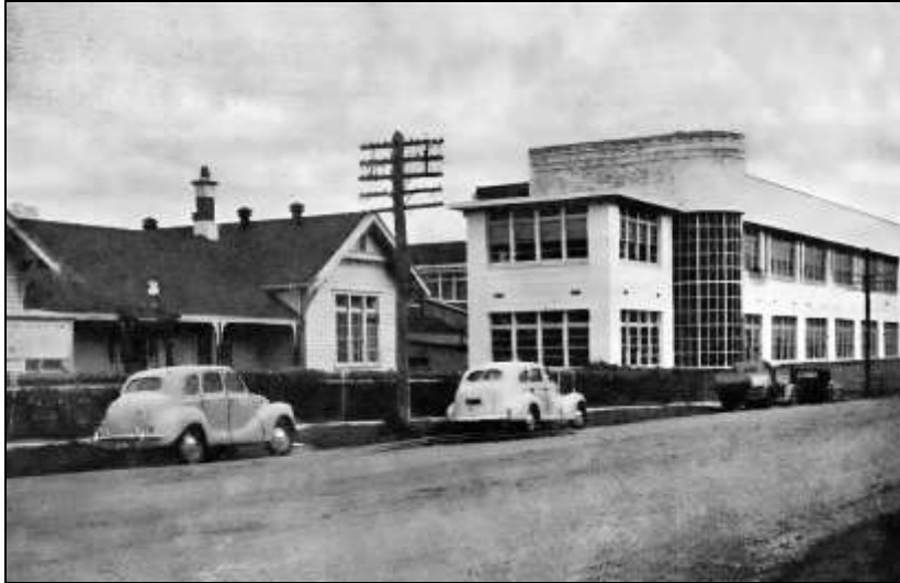
Sunshine Technical School, Office and Engineering Block
