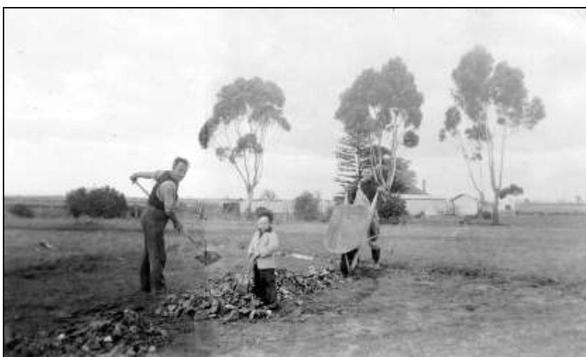
Willy Stein repairing potholes in Walmer Avenue 1930s c/- Mary Smith
