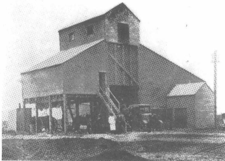
Footscray Council's stone crusher in the 1920s. Crushed rock was raised into the tall hopper above the truck into which it was discharged for road-making sites in the municipality.
