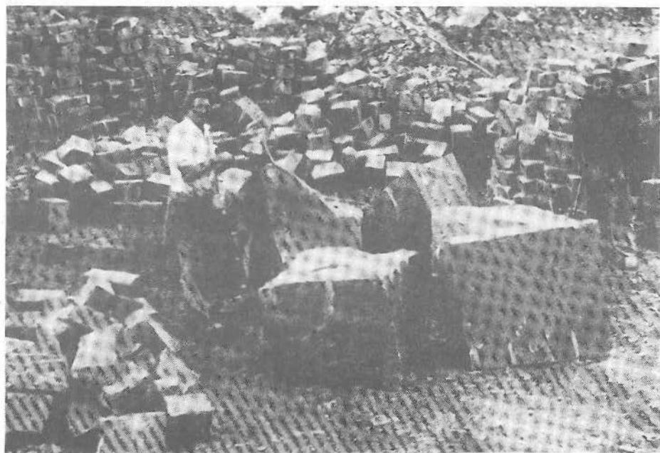
Lords Quarry (later Standard), Brooklyn, in the 1950s. Roughly finished pitchers are stacked in the background behind the large blocks which are being progressively broken down.
