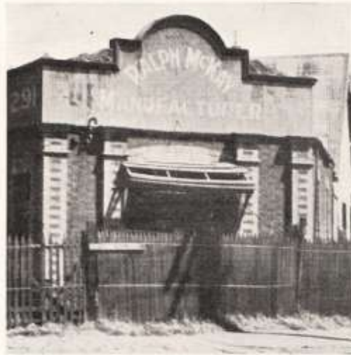
The Original Factory at Ascot Vale.
