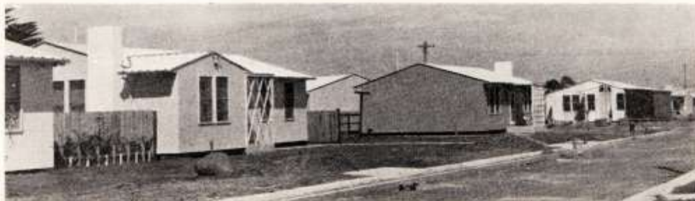
A section of the Railway Homes in course of erection
