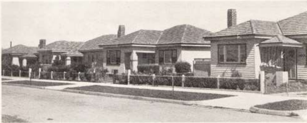
A Good Type of Workmen's Home at Tottenham.
