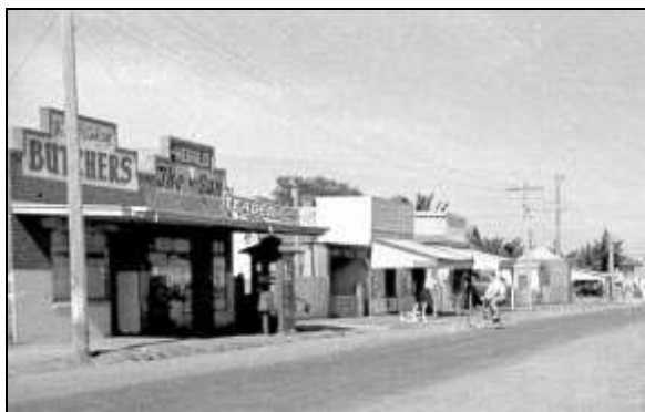
St Albans shopping centre Main Road West 1954
