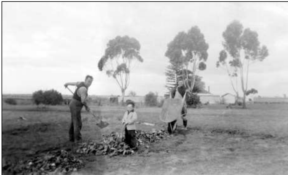
Fred Stein repairing potholes in the road
