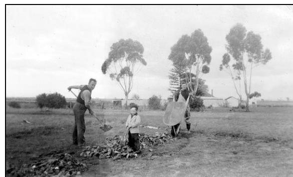
St Albans residents repairing road 1940s © M Smith
