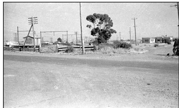
Cnr Mckechnie Street & Main Road West 1955
