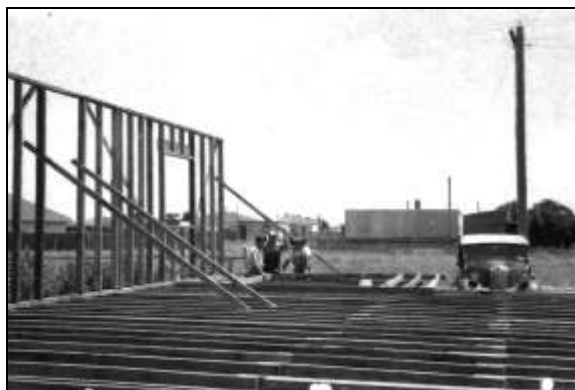
House construction Alfrieda Street © K Haumann
