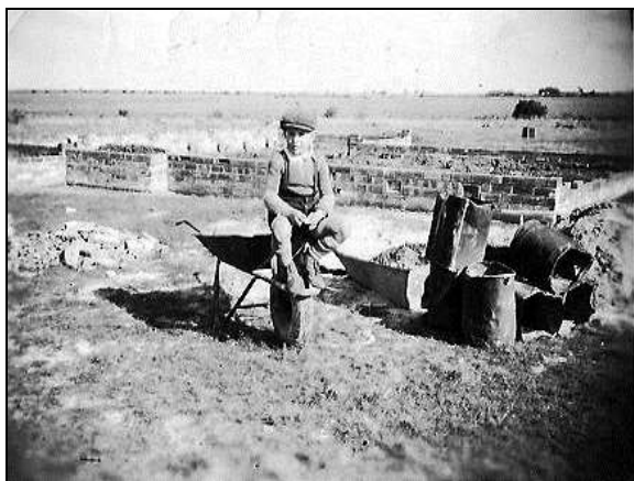
Bernie Kokot on building site 1950s © B Kokot
