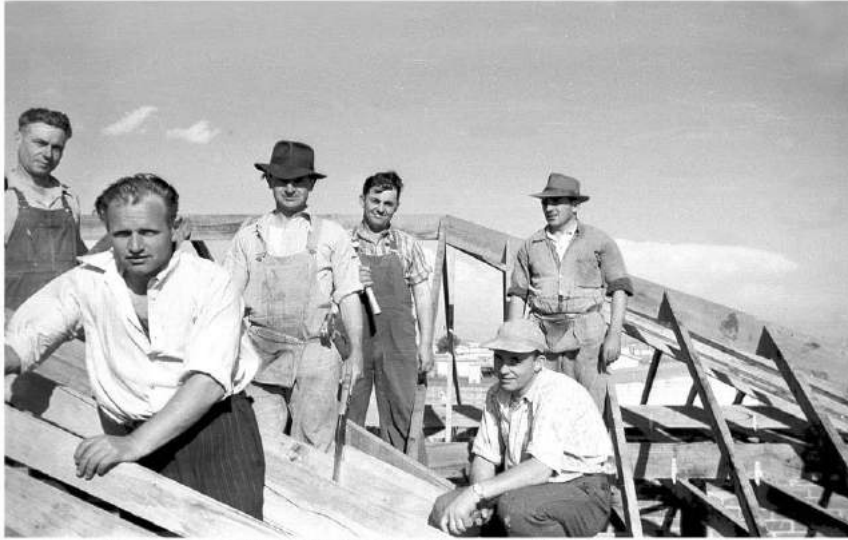
Kon Haumann (front left) and others constructing the roof.
