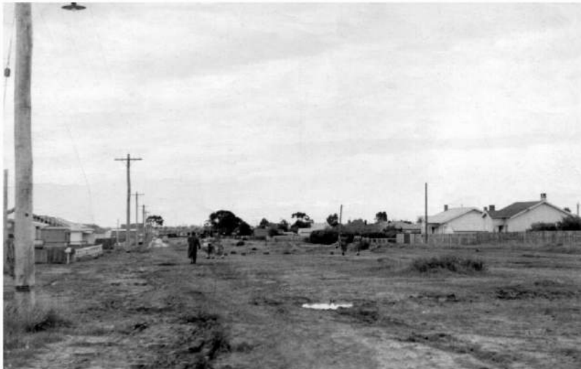
Alfreda Street near Craigielea Avenue looking south, 1955.
