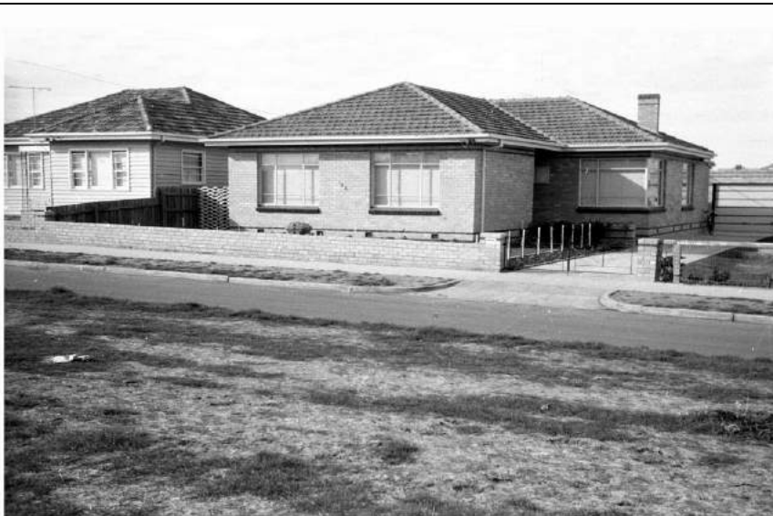
Road and footpath construction, Alfrieda Street, 1957.
