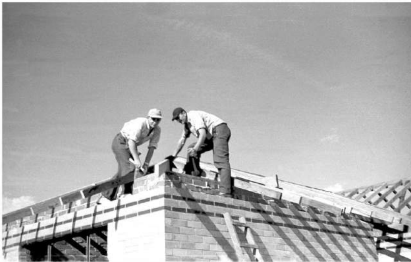
Building the roof, Alfrieda Street St Albans.
