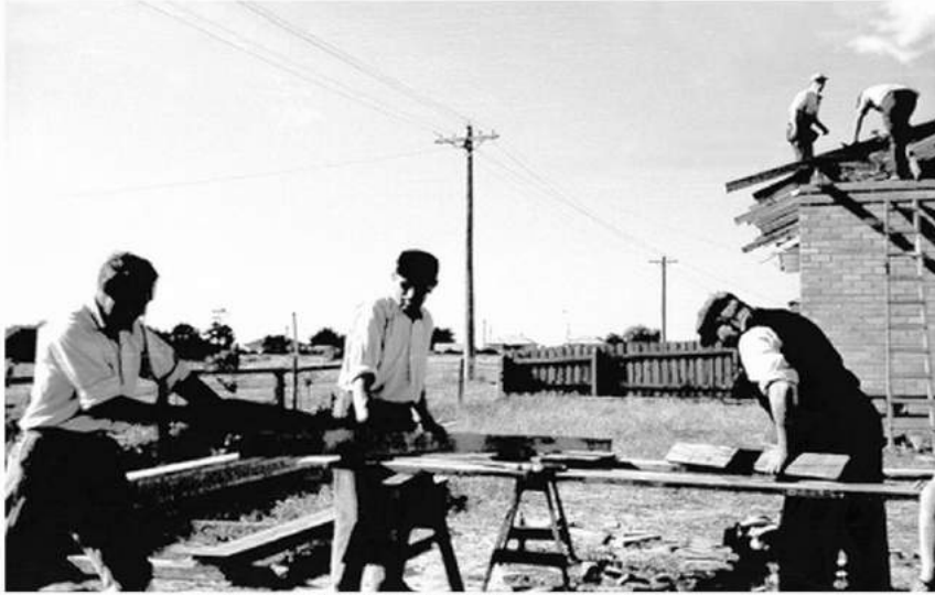
Cutting the rafters for the new house.
